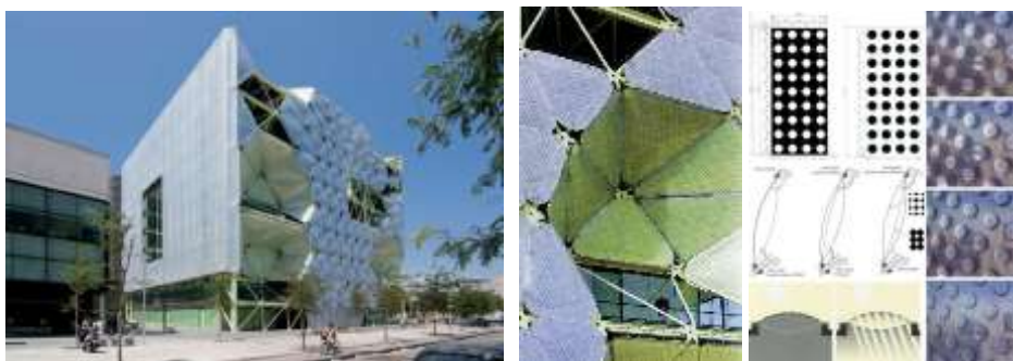
Figure 6: The Media-TIC Building Facade and module detail [URL-8]
