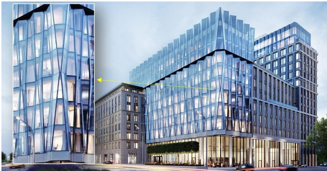
Figure 1. Prismatic Facade Cladding System
