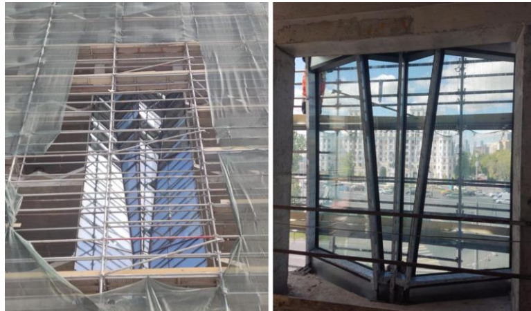
Figure 2. Application of Prismatic Facade Cladding Systems
