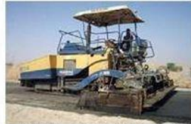
Finisher (Asfalt Serme)
